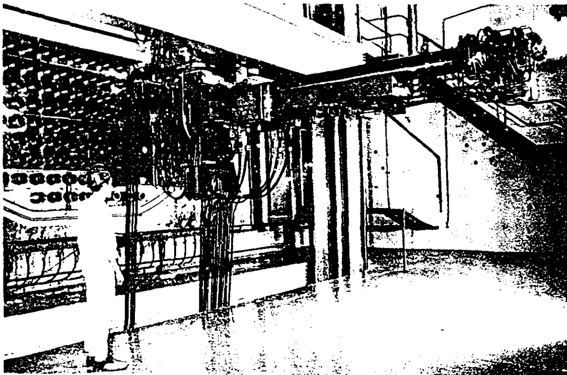
FIGURE 31 Pickering Fuelling Machine
